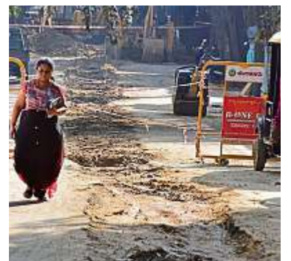
The ongoing road work at Vyalikaval.
